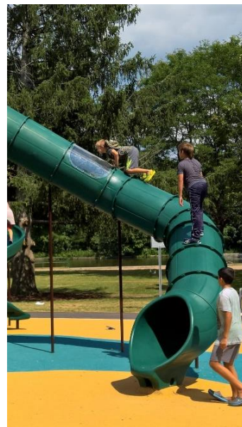
The children use an unintended slide surface to climb and thereby exposing the user to higher fall than intended by the designer
